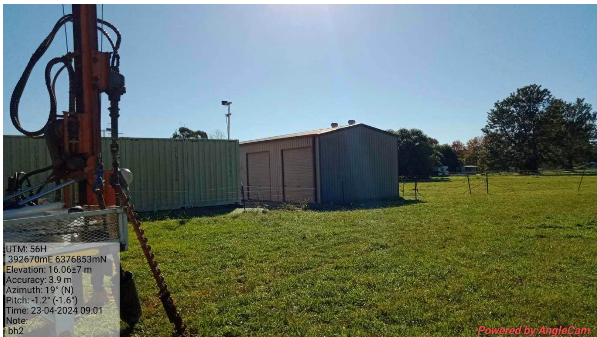
Photograph 6: Location BH02/GW02, facing northeast. Self-storage sheds and containers visible in background (23 April 2024).
